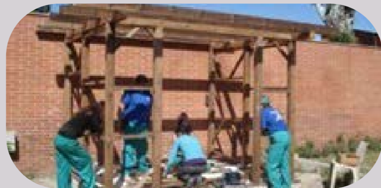
Building the tool shed
