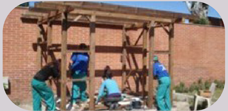
Building the tool shed
